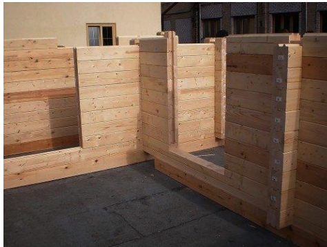
Figure 2. Profiled glue wood beams produced for certain houses
