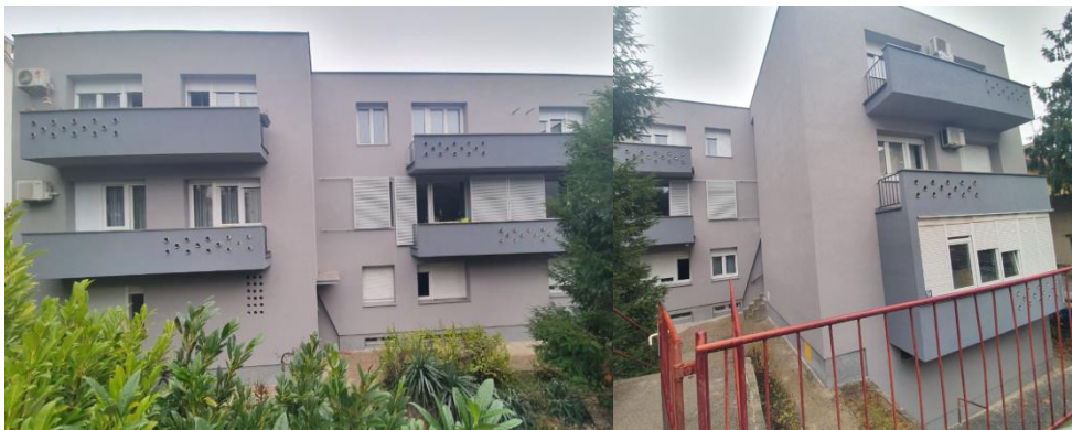
Figure 3: Residential building in Zagreb after energy renovation [3]
