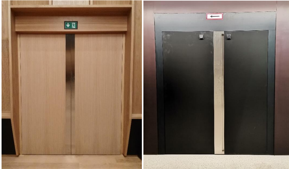
Figure 2: Different surfaces of the doors
