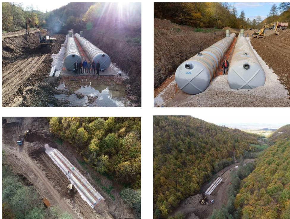
Figure 5: Installation of two tanks with a total volume of 440m 3
