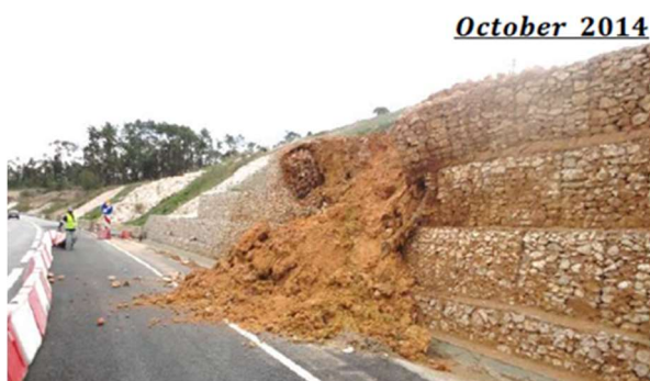
Figure 5. Damage to the gabion wall [11].
