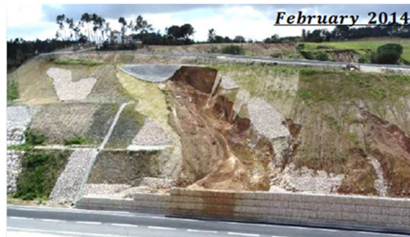
Figure 4. Sliding due to heavy rain [11].
